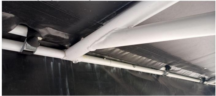
\*Canopy straps & bolts must be retightened after 2-3 days!\*
